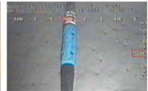
Figure 3. As shot from the remotely operated vehicle, the four-component cable as it looks on the seafloor. (Photo courtesy of Multiwave Geophysical)
